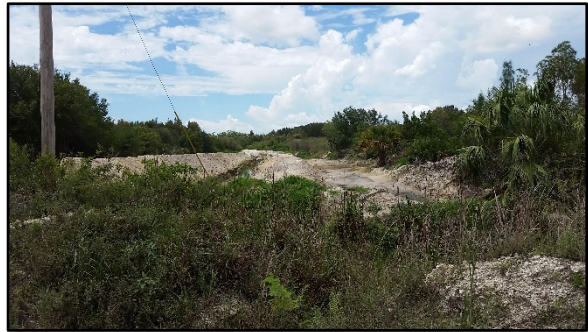
E) Western perimeter rim ditch
