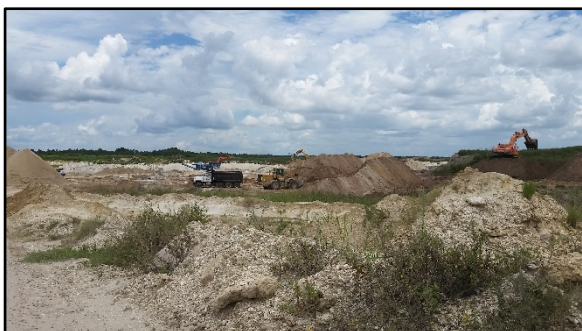
D) Fill dirt operation
