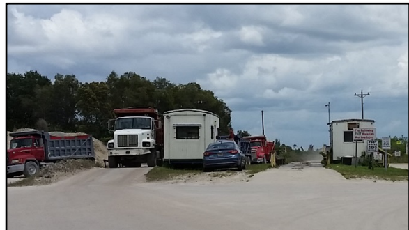
A) Scales and scale houses (trailers)
