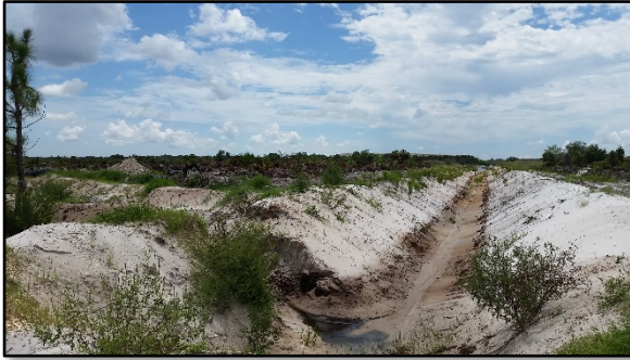
E) Northern rim ditch for new excavation
