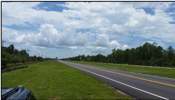
B) Southbound US Hwy 41 from SW corner
