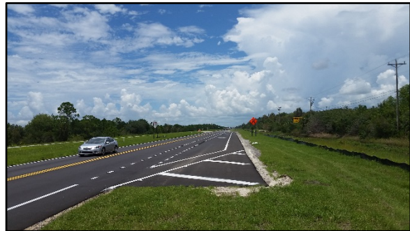
B) Northbound US Hwy41 from SW corner
